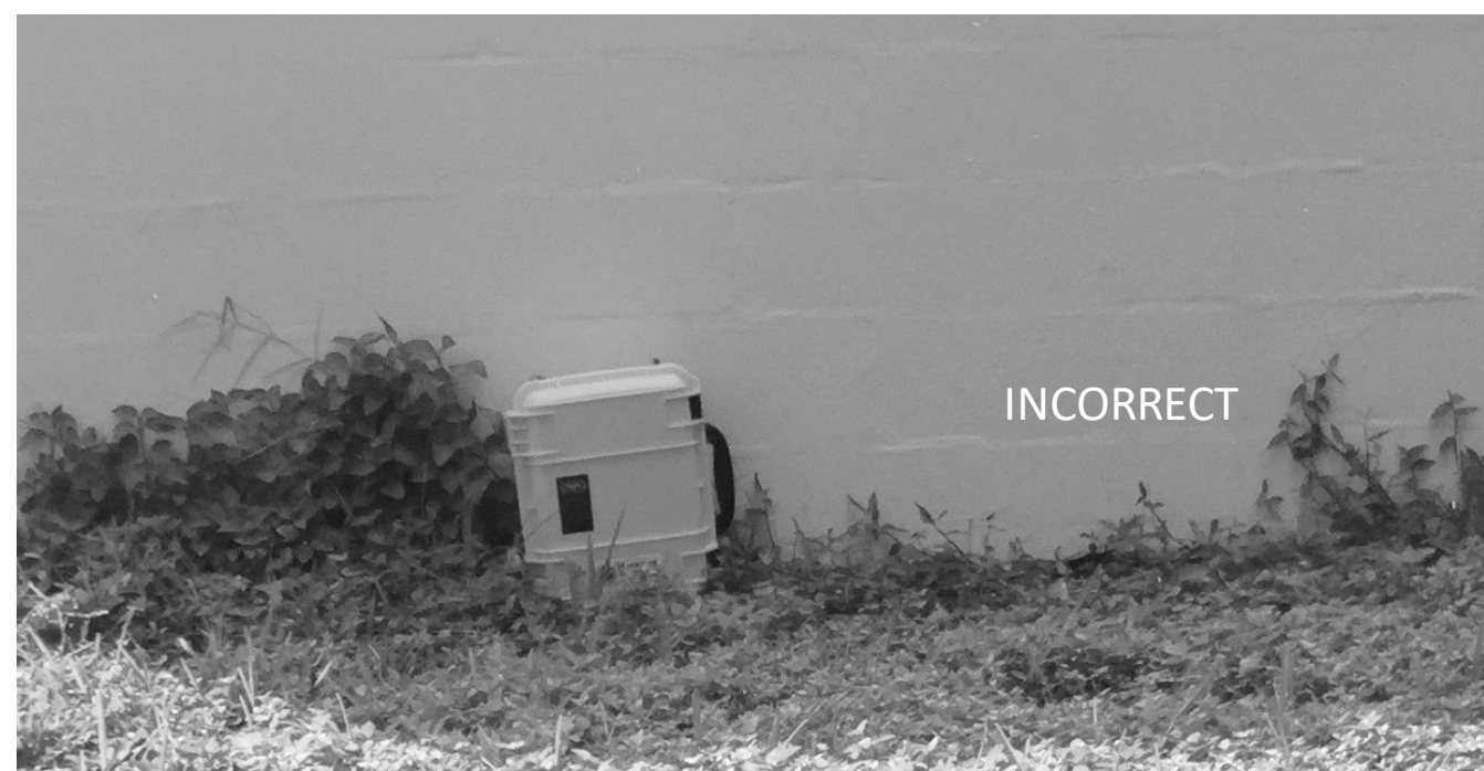
FIGURE 3-14 sensor too close to a cinder block wall.
