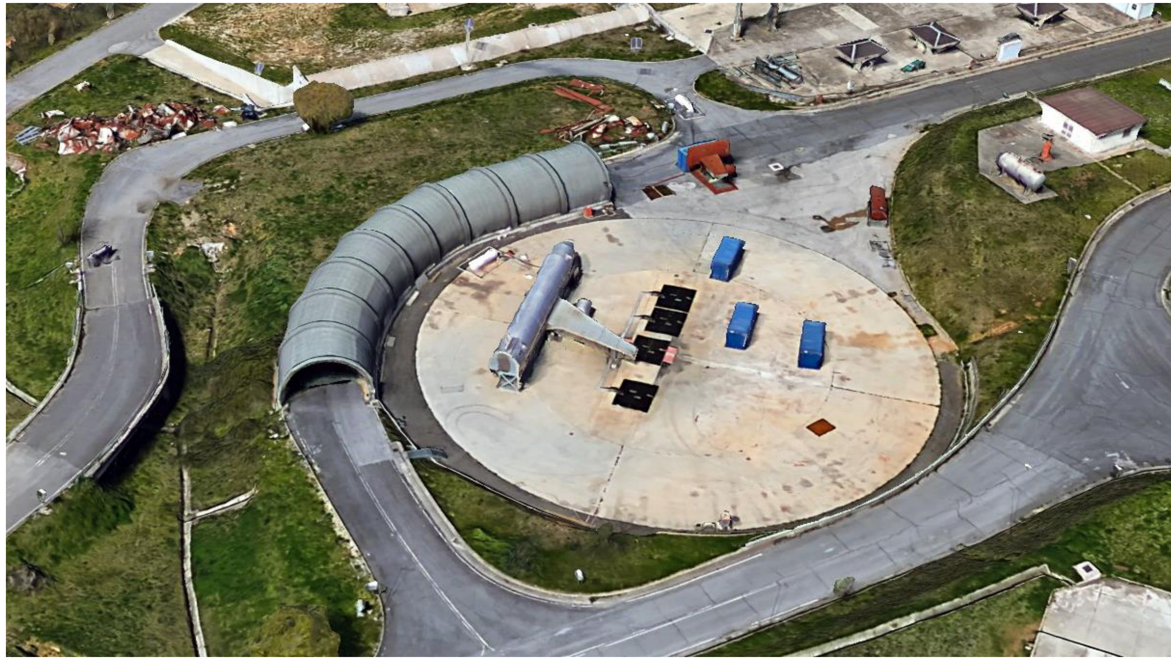
Scuola Di Formazione, Montelibrettese, Italy. National Search and Rescue Training Center.
