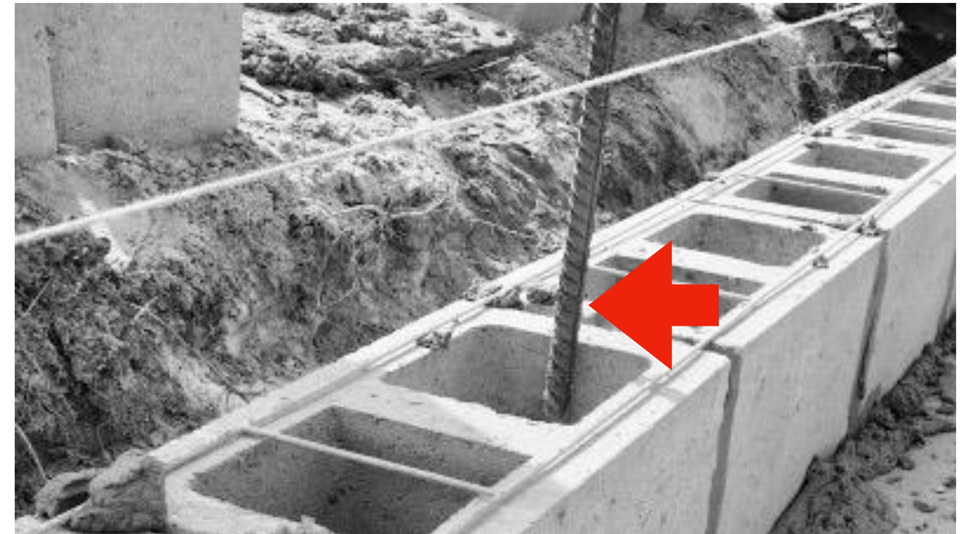
FIGURE 3-1 Rebar reinforced cinder block.
