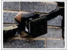
Once the ratchet is tightened, place a wedge or piece of wood, behind the plate to create a stable platform.
